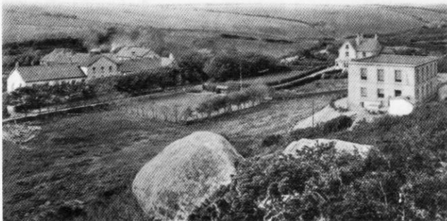
Porthcurnow cable station and offices in 1909
